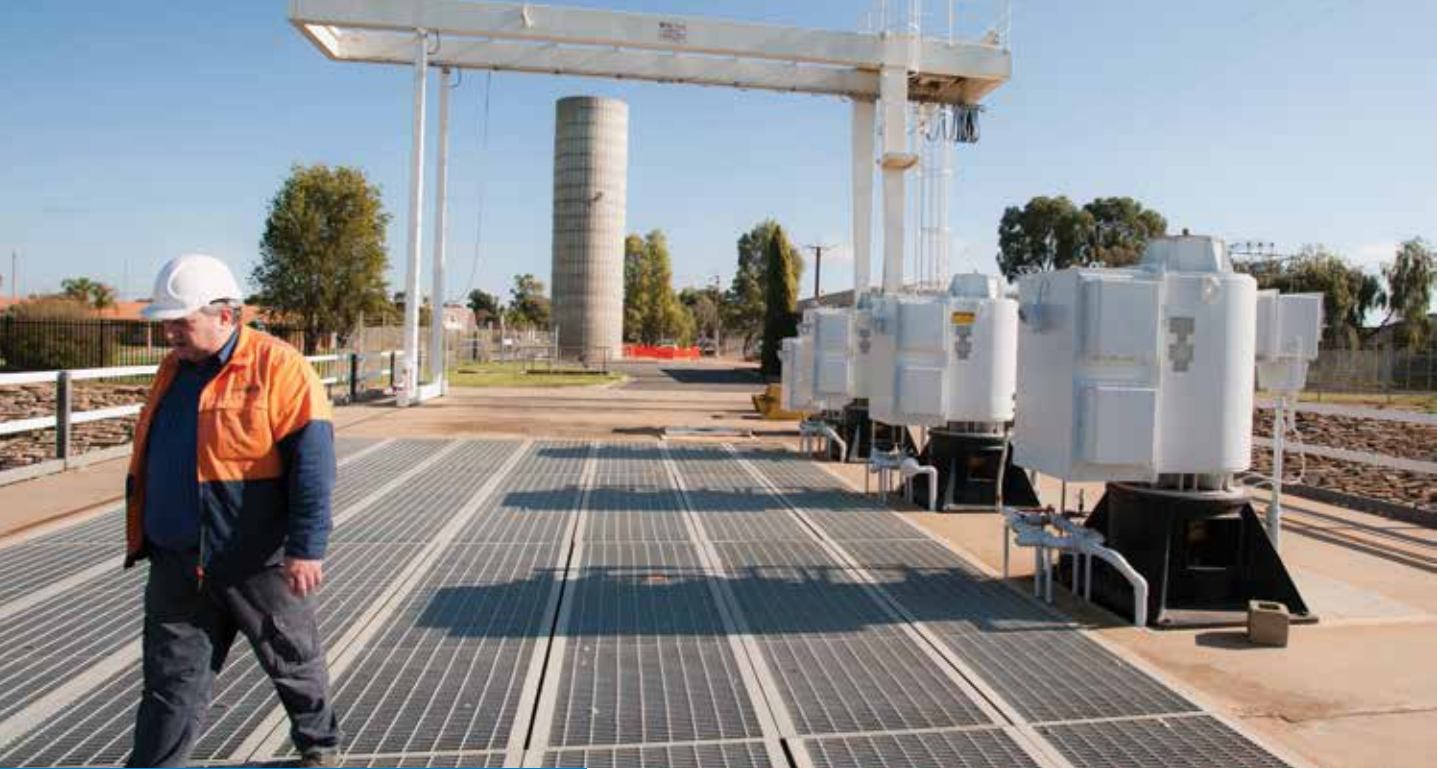
Renmark Irrigation Trust Pump Station, Renmark
