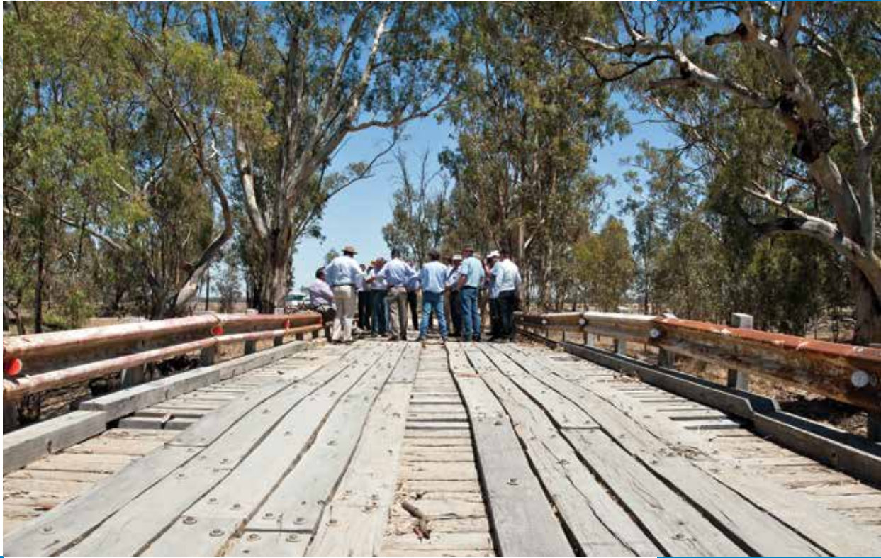
Sandy Creek Bridge, Barber Creek, Barham
